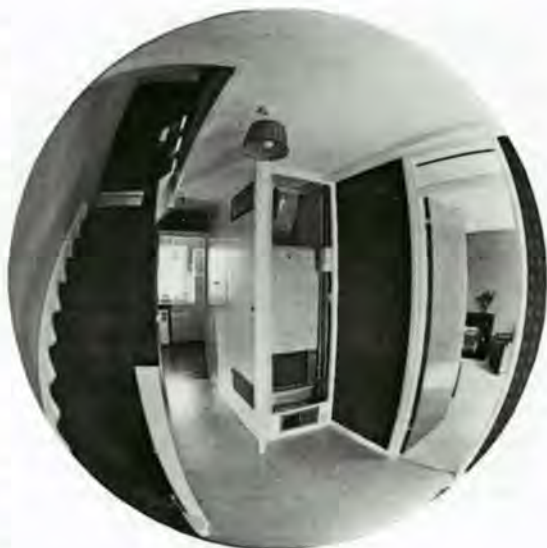
This 'fish-eye' picture is of an all-electric house on a new estate. An eight kilowatt Creda Electricaire unit sited in the hall provides ducted warm air heating to the lounge/dining room, hall and two bedrooms. An electric furniture unit fire makes a pleasing focal point in the lounge.
